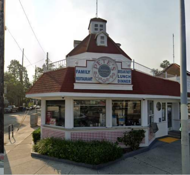
1 2400 HOOVER ST SETBACK: 0' (ZIMAS) # STORIES: 1 HEIGHT: 12' (PERMIT) MATERIAL: BRICK COMMERCIAL VERNACULAR COMMERCIAL BUILDING
