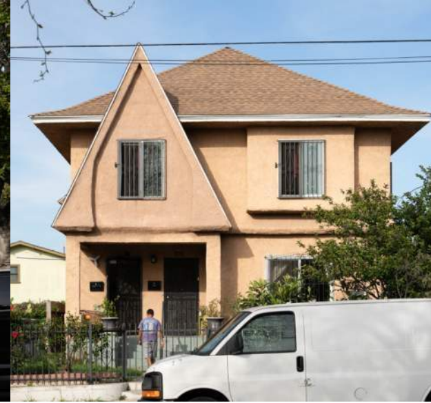
14 1037 W 22ND ST SETBACK: 14' (ZIMAS) # STORIES: 2 ESTIMATED HEIGHT: 26' MATERIAL: STUCCO PROVINCIAL REVIVAL RESIDENTIAL
