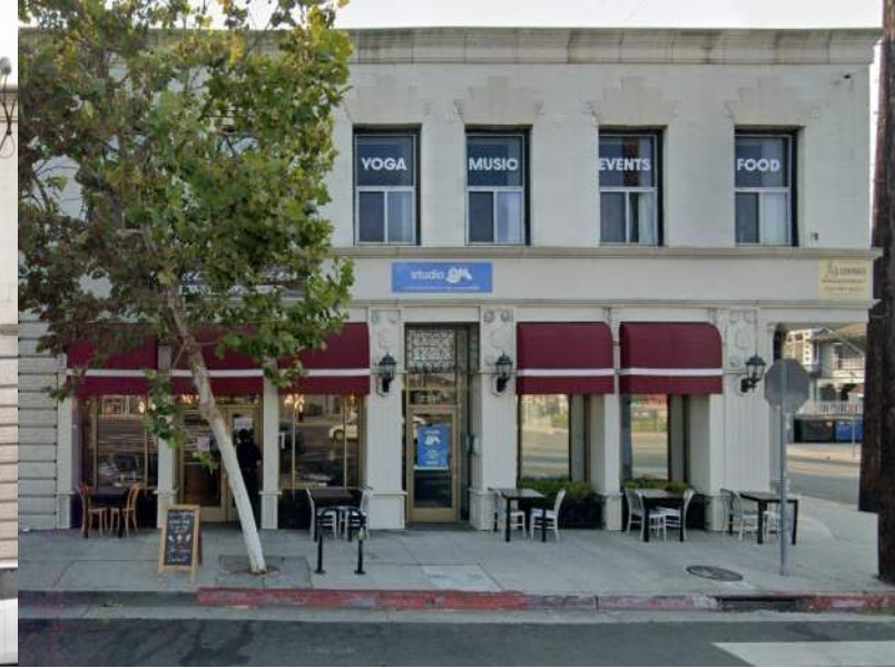
2 2316 UNION AVE SETBACK: 0' (ZIMAS) # STORIES: 2 HEIGHT: 23' (PERMIT) MATERIAL: BRICK COMMERCIAL VERNACULAR COMMERCIAL BUILDING
