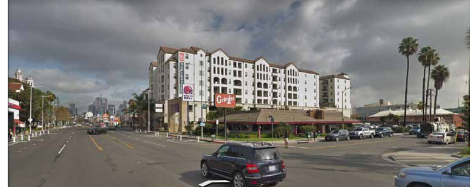
S FIGUEROA STREET, LOOKING AT SITE
