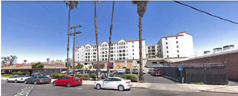
W 28TH STREET, LOOKING AT SITE
