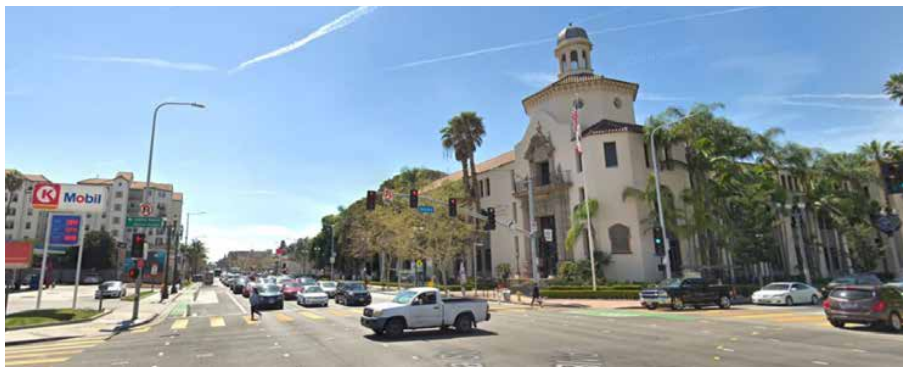
S FIGUEROA STREET AND W ADAMS BLVD, LOOKING AT AAA BUILDING
