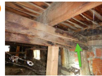
split floor beam
